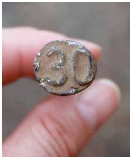
(Above) Date nails, such as this one from 1930, were used by railroads to identify the age of a tie. (Right) The elevators at Willada.
