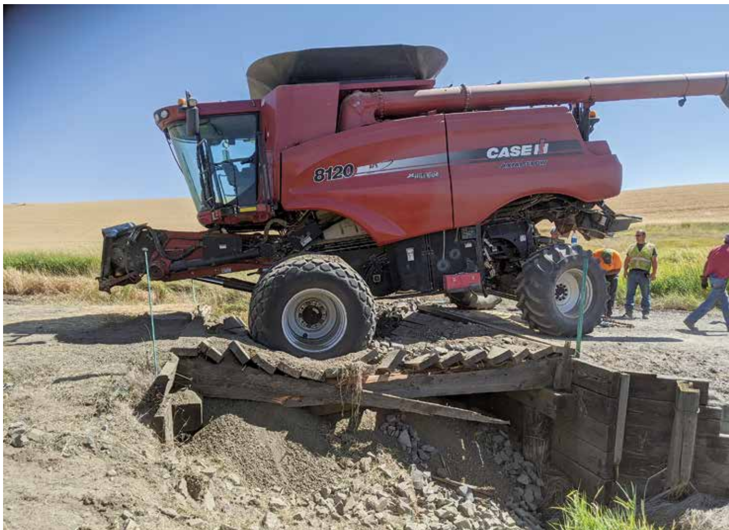
Older, shorter-span bridges weren't built for today's modern farming equipment, which is becoming heavier and wider. County officials are warning farmers to take precautions before moving farm equipment across county structures, such as emptying tanks, removing headers, or avoiding structures whenever possible. Even newer bridges are susceptible to failure if load limits are exceeded. Photo courtesy of the Whitman County Public Works Department.
