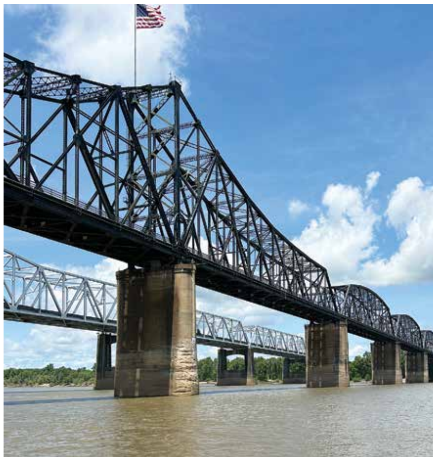
The piles on the Old Vicksburg Bridge shows evidence of past vessel collisions. You can watch real-time traffic through this stretch of the Mississippi River by googling "earthcam Vicksburg."
