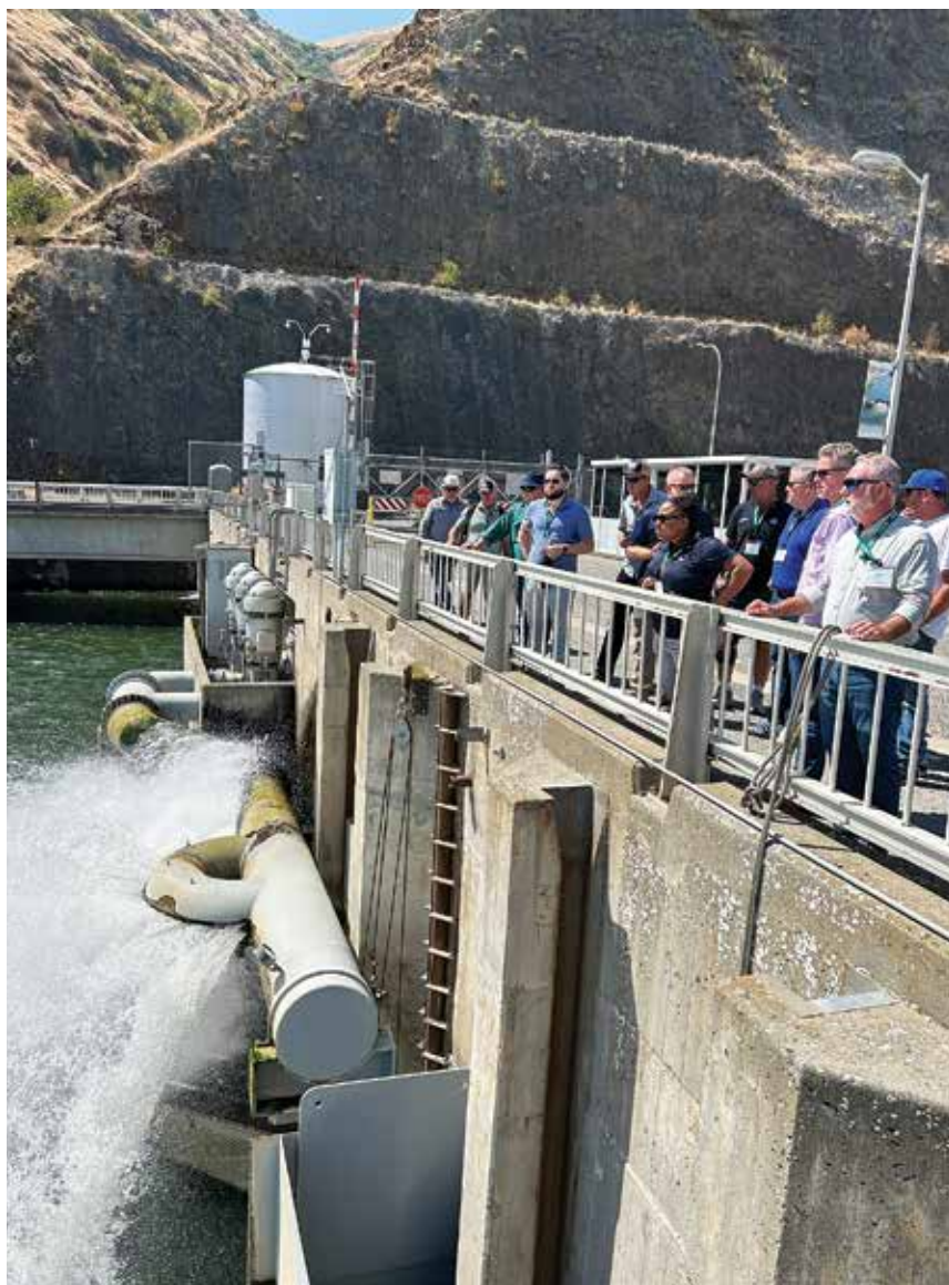
One of the highlights of the tour of Lower Granite Dam was learning about the efforts that have been put into the fish passage system, such as this cooling tower that brings up cold water from the base of the dam to help keep surface temperatures cooler.
